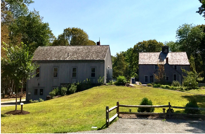
Alden Homestead Duxbury
