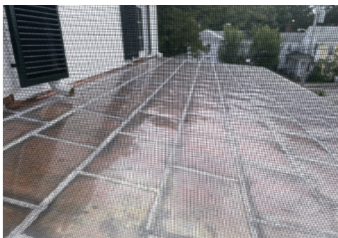
View of copper roof
